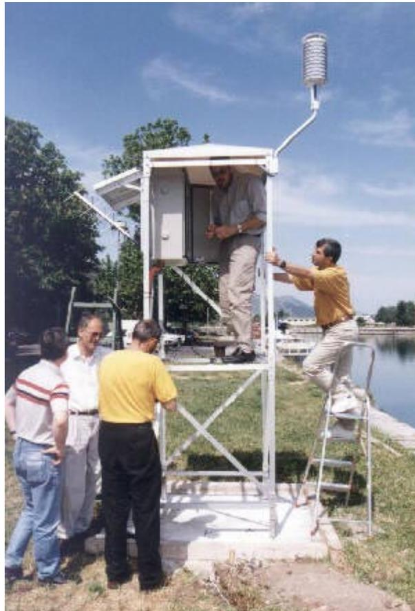
Installation of a hydrometeorological data collecting platform in Croatia
